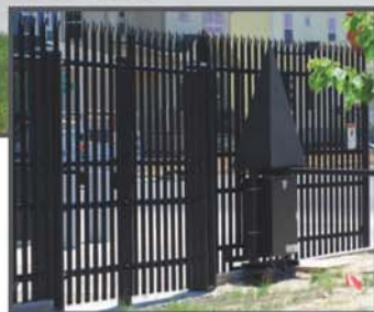
The main gate entrance and guard shack at the Denver regional office of the FBI. At right, a gate and gate operator typical of the high security installation.
